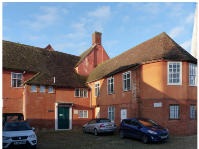
Figure 34: Assembly Room and stair outshot from SE (CAL).
