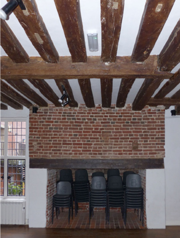
Figure 12: Guildhall GF- cross passage evidence from E, stair trap to right (CAL).
