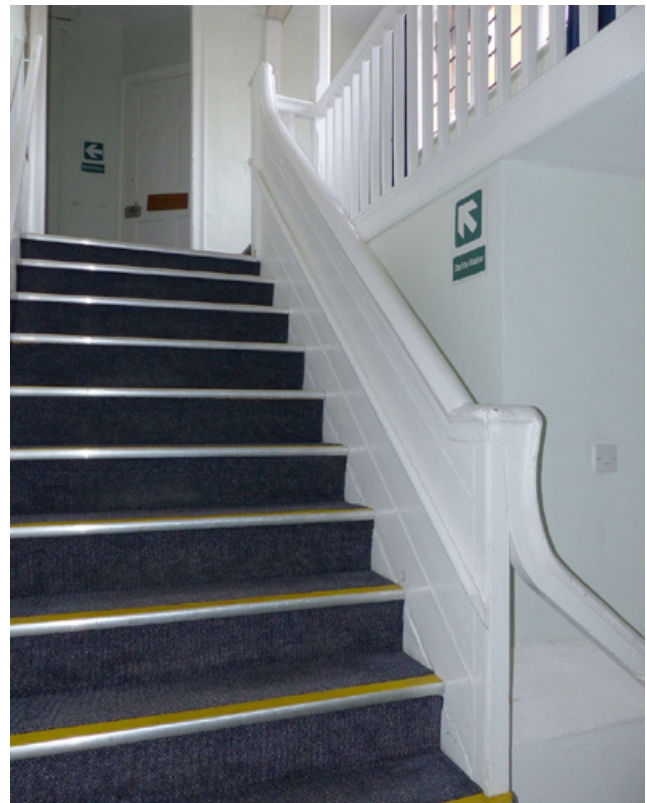
Figure 36: Assembly Room stair (CAL).
