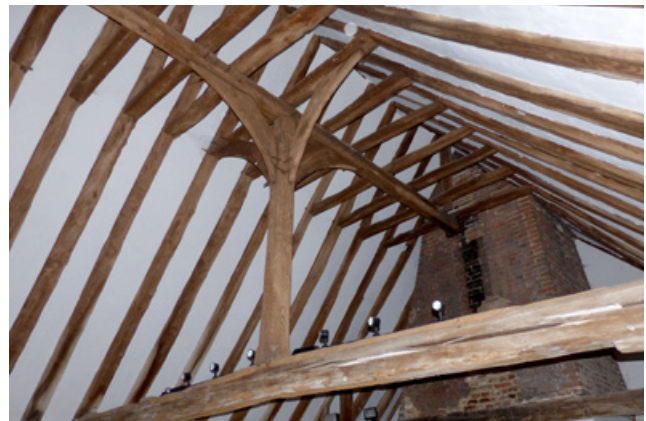
Figure 26: Market Hall 2F- crown-post roof from SW (CAL).
