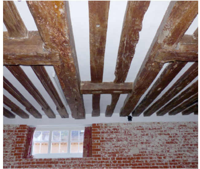
Figure 13: Guildhall GF- stair trap from W (CAL).
