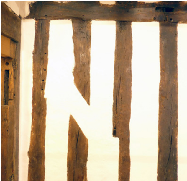
Figure 29: Market Hall GF- blocked doorway, possible evidence for porch (CAL).
