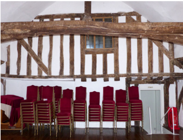
Figure 16: Guildhall 1F showing south elevation of Market Hall (2F) (CAL).
