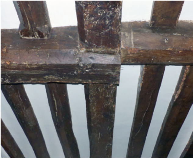
Figure 14: Guildhall GF- original N end, extension to R (CAL).
