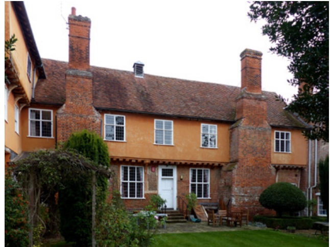
Figure 8: Guildhall from W, stair block to left (CAL).
