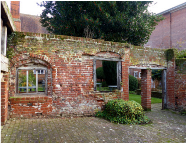
Figure 31: Kitchen interior from W (CAL).
