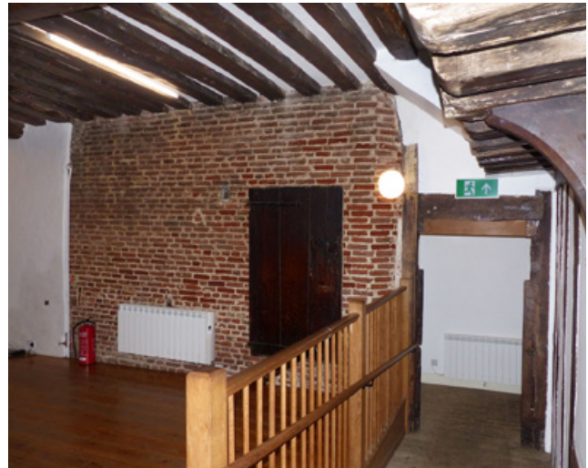
Figure 17: Guildhall extension GF- junction with Market Hall (CAL).
