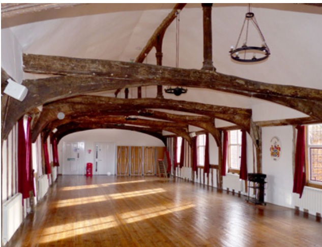
Figure 15: Guildhall 1F crown-post roof from NE (CAL).
