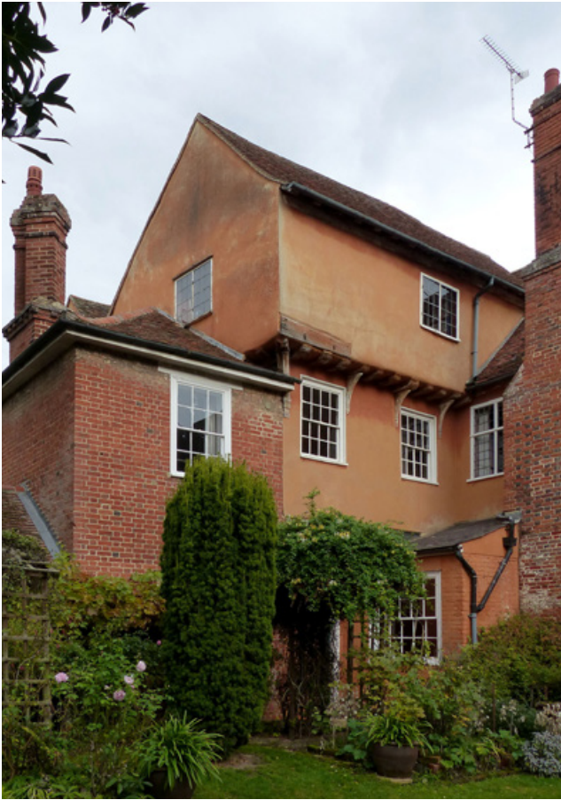
Figure 27: Stair block from SW (CAL).
