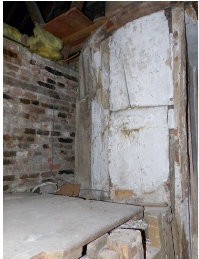
Figure 30: Stair block- perimeter of stair (CAL).
