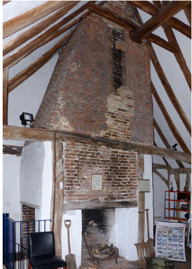
Figure 25: Market Hall 2F – inserted stack (CAL).
