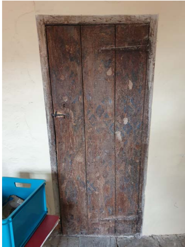
Photograph 57 – Historic timber plank door providing access to ‘C7’
