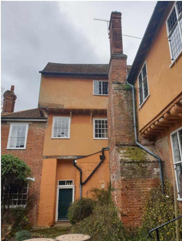
Photograph 40 – Part of the south elevation of the middle range, as seen from the courtyard
