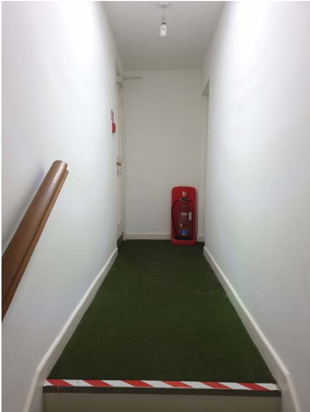
Photograph 103 – Hallway built within 'L1' leading to 'R10' kitchenette
