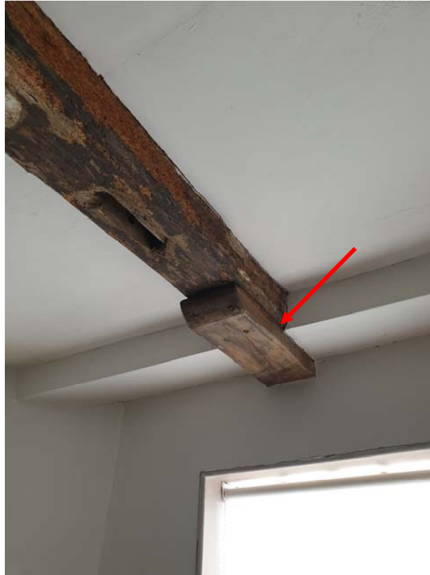
Photograph 71 – Improved bearing of the beam over 'R6' at the east end
