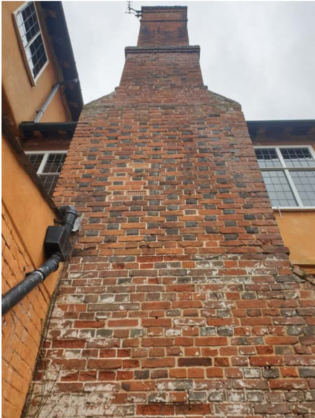
Photograph 93 – West elevation of the Old Town Hall's north chimney
