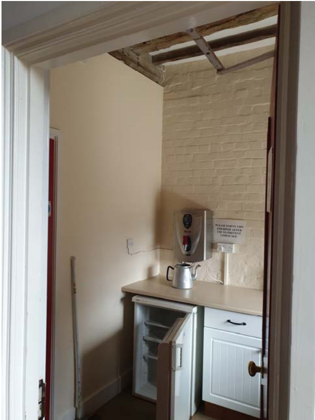
Photograph 112 – Room 'L7' looking south-east
