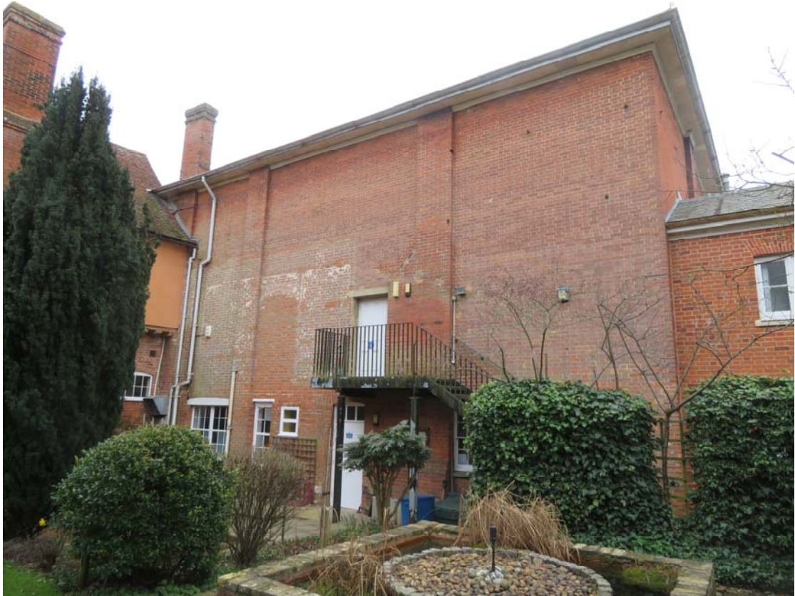
Photograph 128 – North elevation of the New Town Hall
