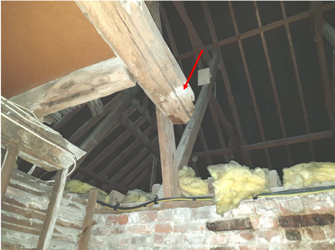
Photograph 59 – Cut back historic timber frame within room 'C7'
