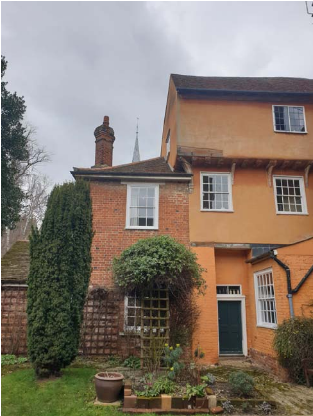
Photograph 17 – South elevation of Caretaker's range
