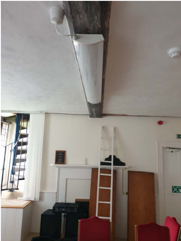
Photograph 60 – Room 'R5' looking east
