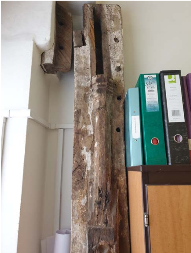
Photograph 78 - Original timber-frame post in 'R8'
