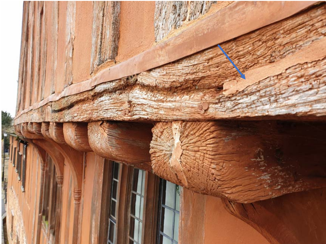
Photograph 31 – Plastic repairs to decayed soleplate of the middle range
