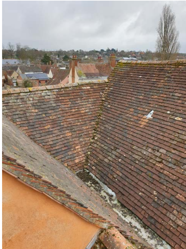
Photograph 23 – Roof arrangement over the Market Hall's middle range
