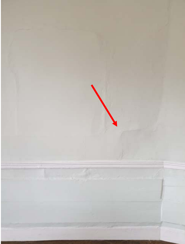
Photograph 65 – Live plaster to the walls noted in 'R1'
