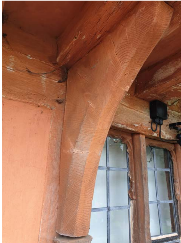
Photograph 35 – Jetty brackets generally found in good condition
