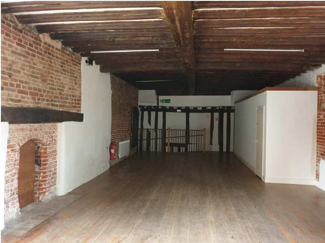
Photograph 106 - Room 'L4' looking north
