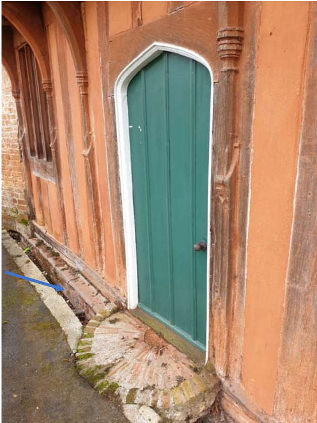
Photograph 38 – Existing ditch along the perimeter of the North elevation (middle range)
