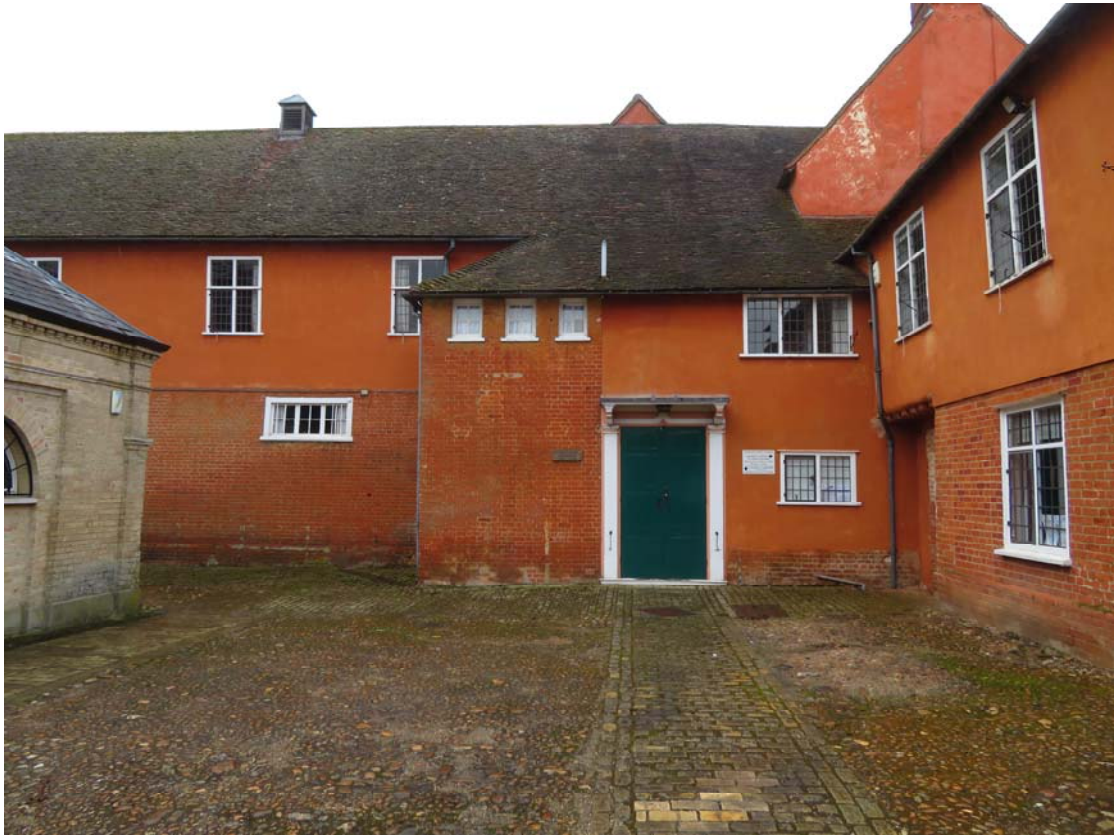
Photograph 100 – Main access into the Guildhall (east elevation)
