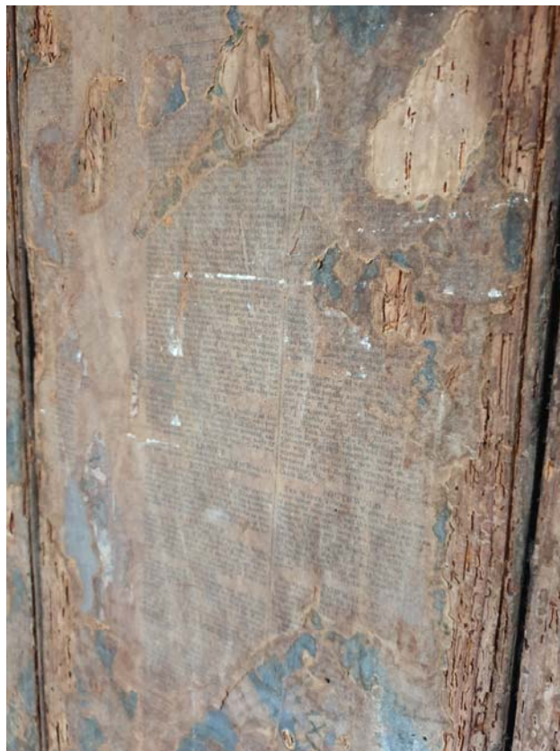
Photograph 58 – Historic newspaper marks on the timber plank door to ‘C7’
