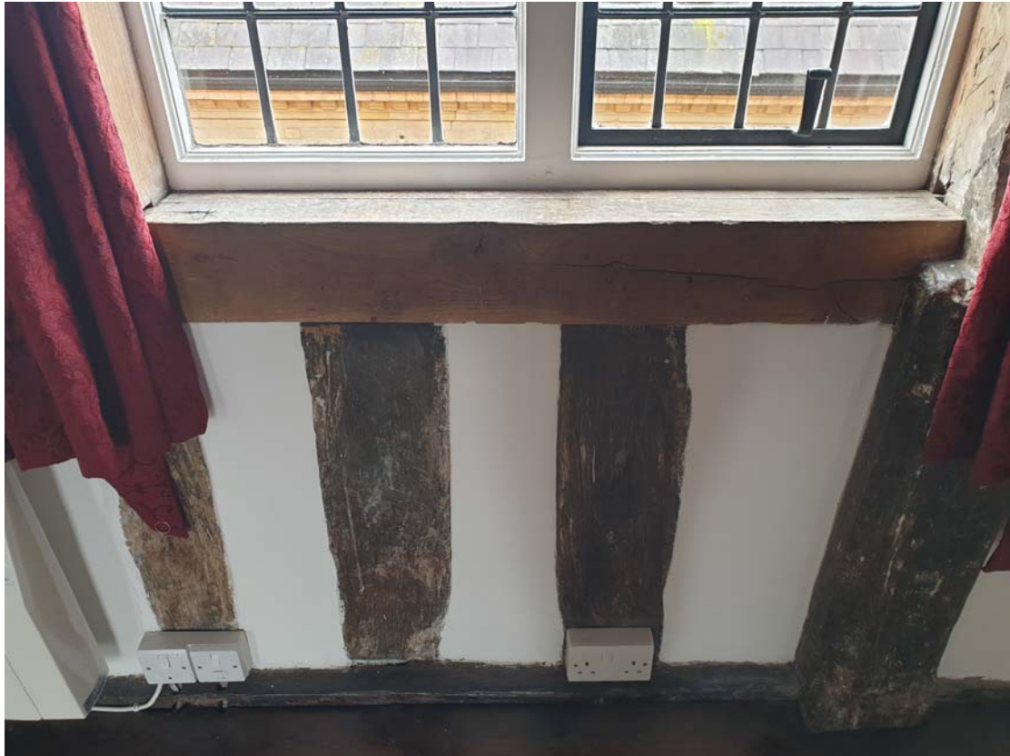
Photograph 115 – Timber sill replacement noted to most of the windows in 'L1'
