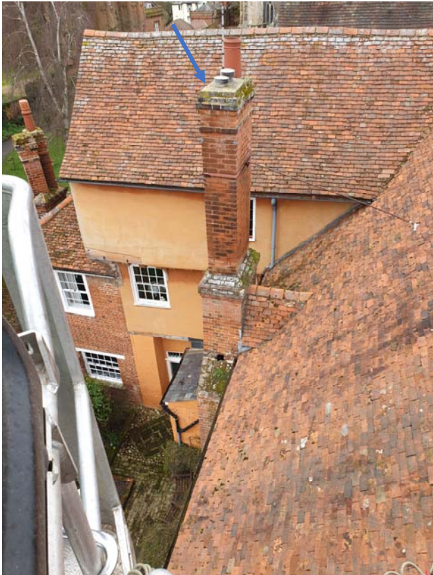
Photograph 87 – North chimney of the Old Town Hall
