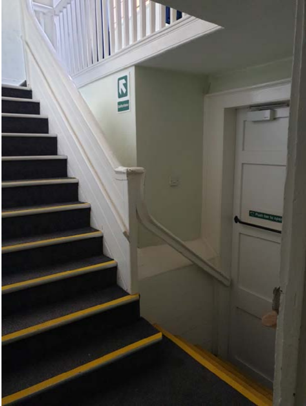
Photograph 101 - Main access into the Guildhall, as seen from inside
