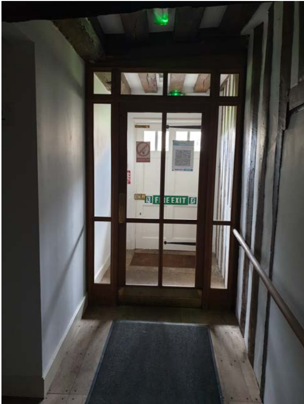
Photograph 69 - Recently re-decorated hallway ('L11')
