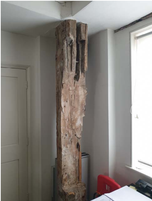
Photograph 76 – Original timber-frame post in 'R7'
