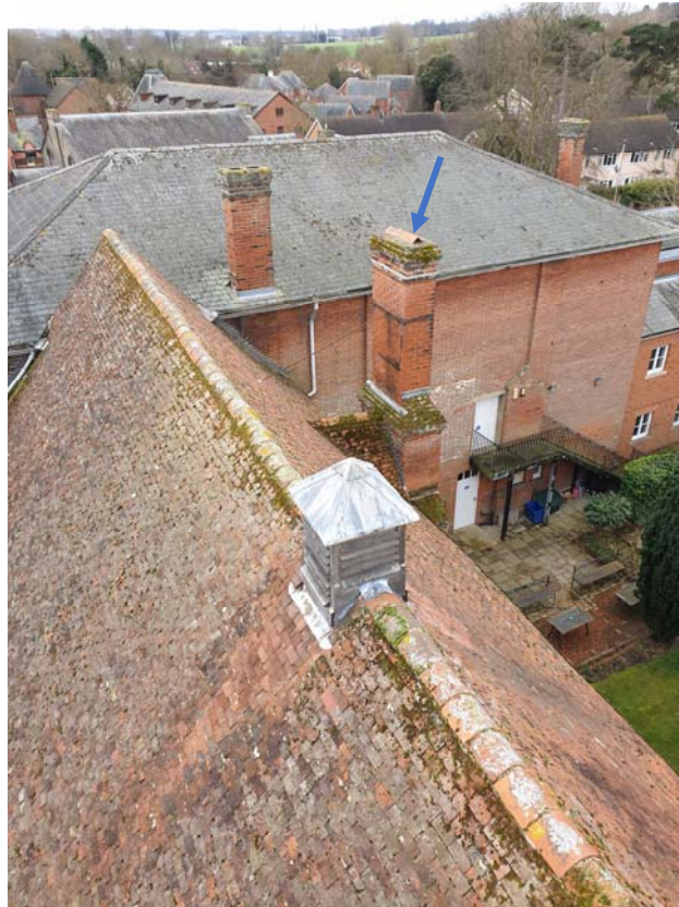
Photograph 89 - South chimney of the Old Town Hall
