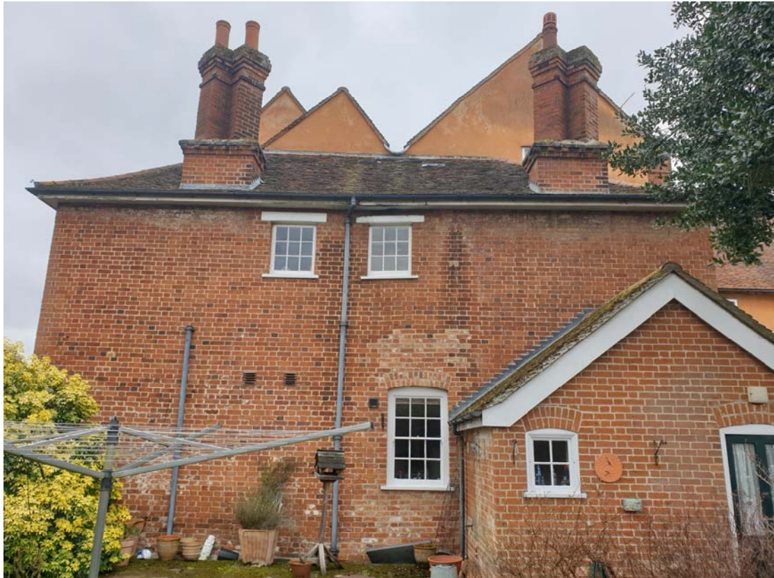
Photograph 13 – West elevation of Market Hall's west wing
