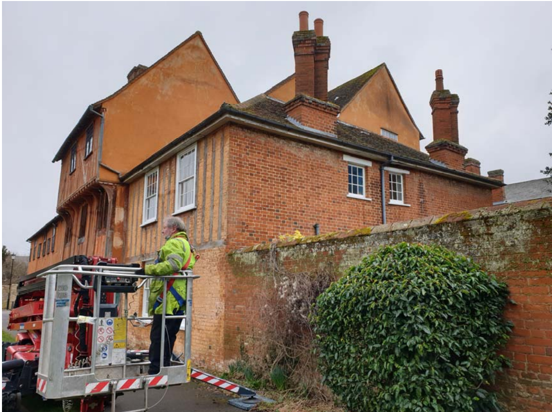
Photograph 01 – Market Hall’s west section
