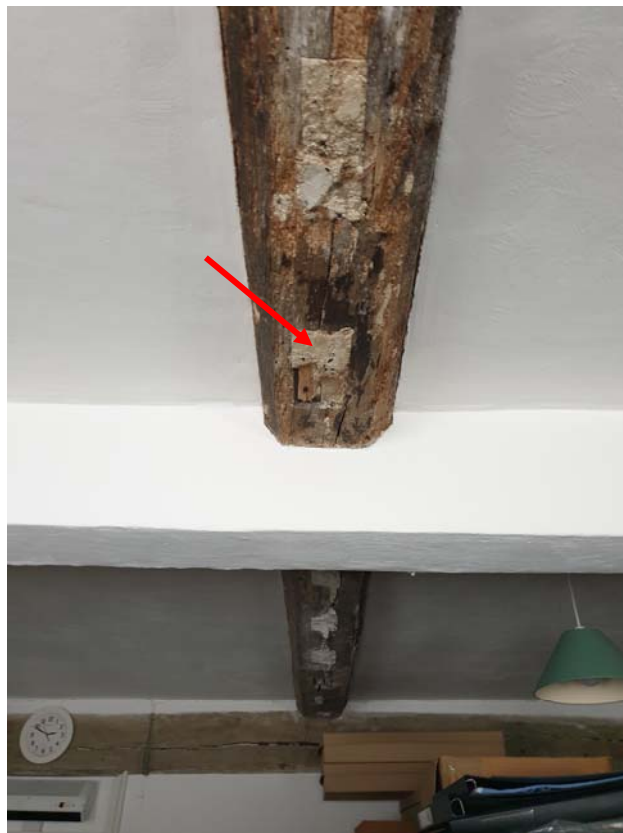
Photograph 72 – Filled mortises to the soffit of the beam over 'R6'
