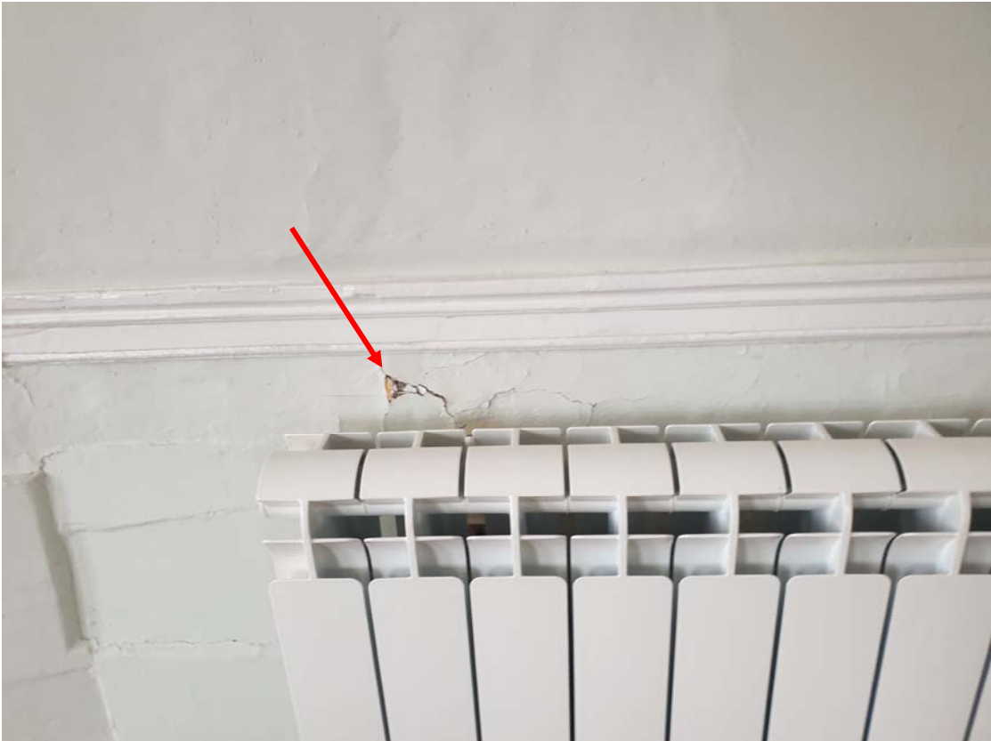
Photograph 66 - Live plaster to the walls noted in 'R1'
