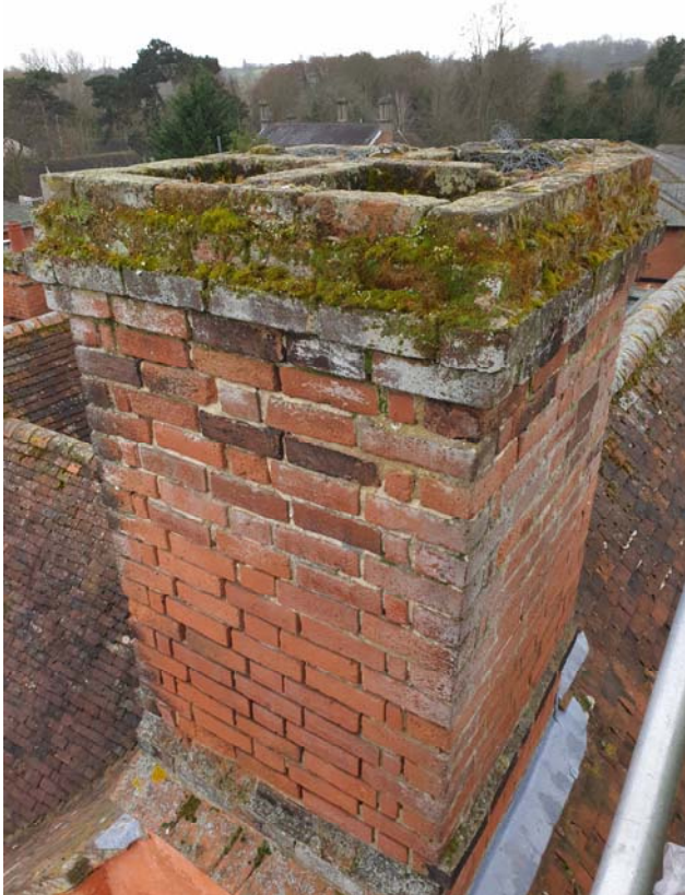
Photograph 19 – Chimney stack to the Market Hall’s middle range
