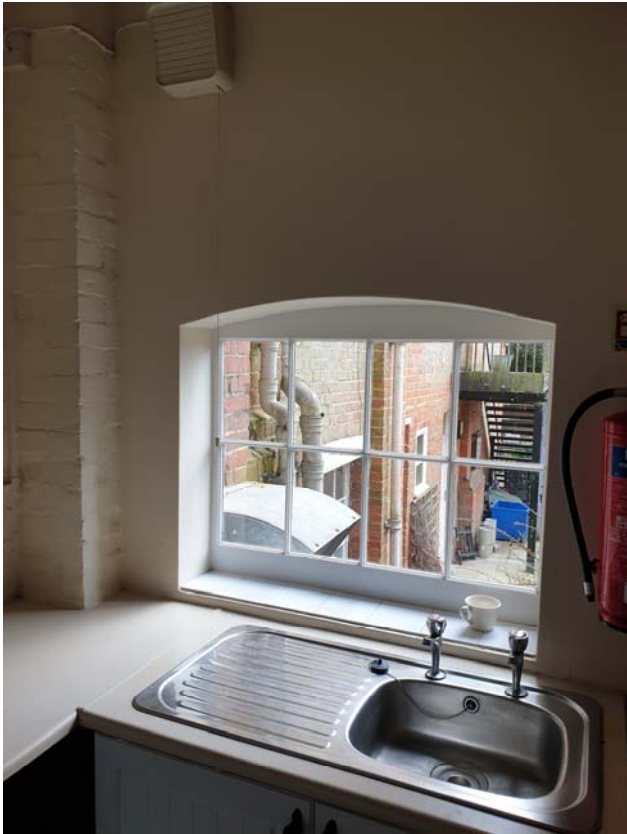
Photograph 111 – Room 'L7' looking west
