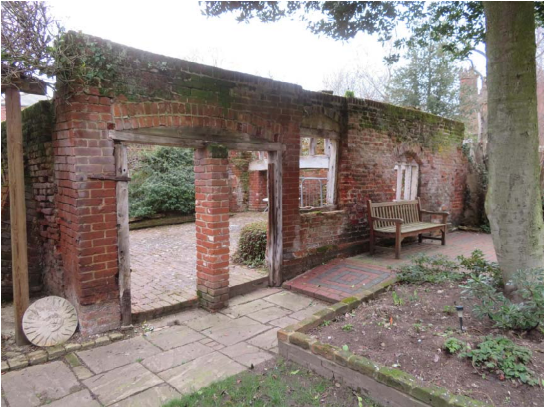
Photograph 132 – The old Tudor kitchen, as seen from the back courtyard
