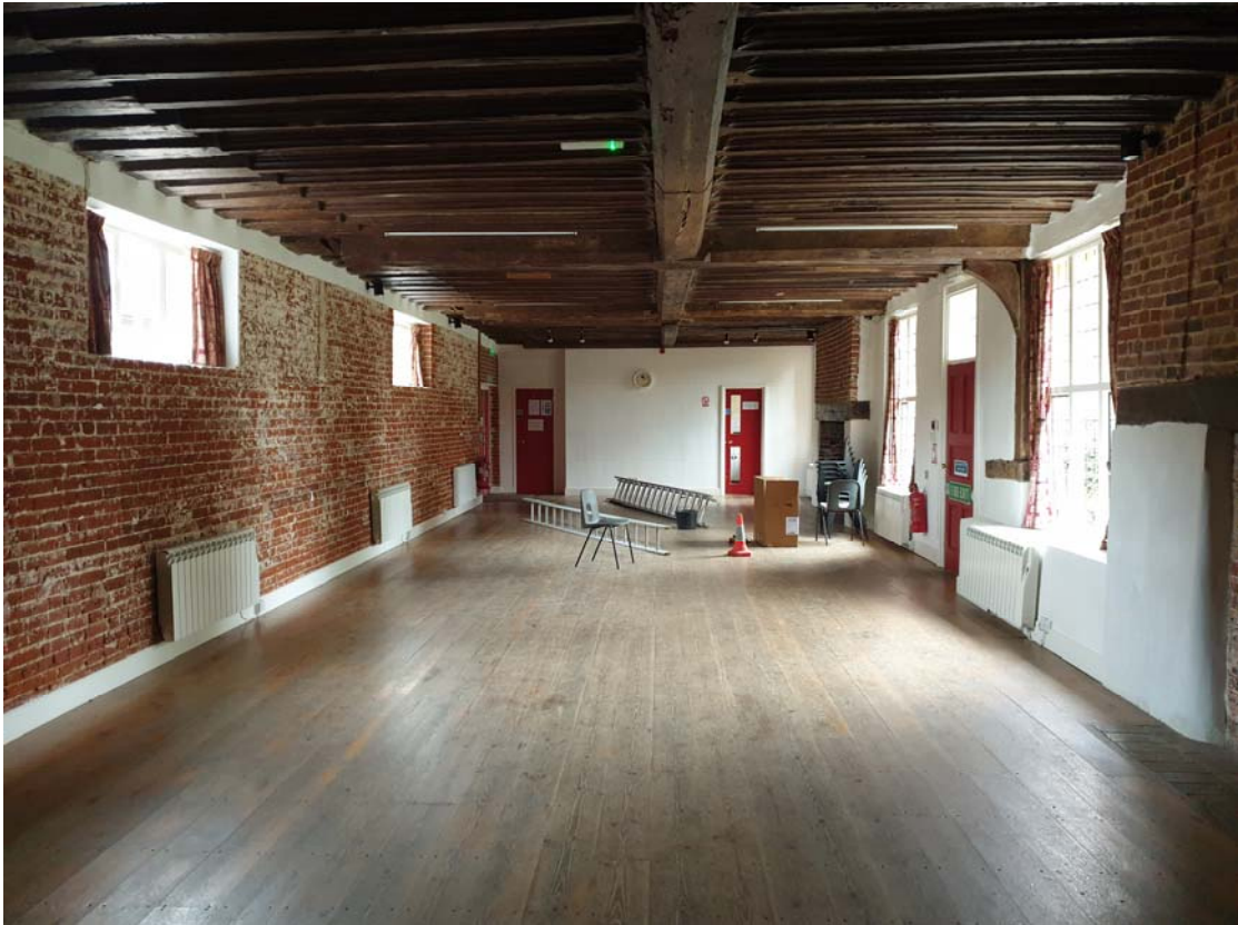
Photograph 105 – Room 'L4' looking south
