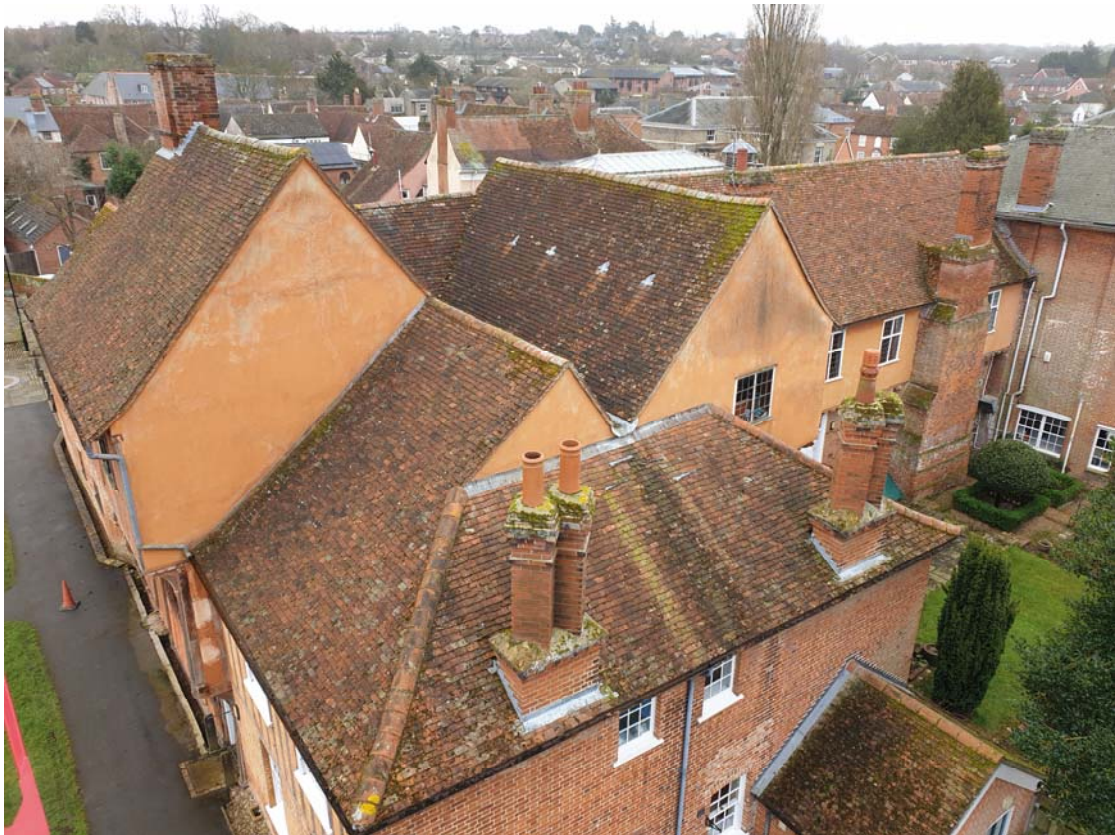
Photograph 02 – Market Hall and Old Town Hall roofs, as seen from the cherry picker
