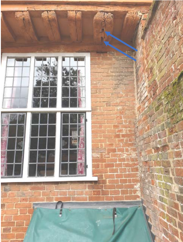
Photograph 95 – Historic mortices indicating a different structural arrangement
