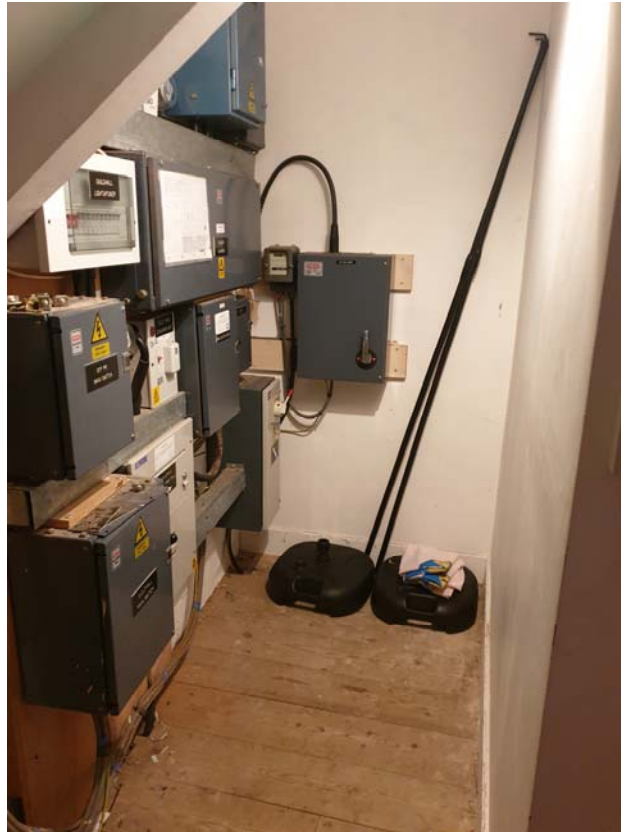
Photograph 113 – Electrical room adjacent to 'L7'
