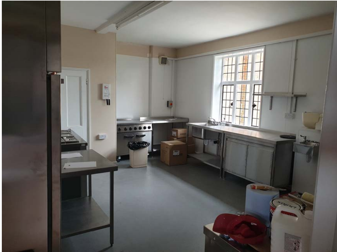
Photograph 117 – Existing kitchen to the south end of room 'L1'
