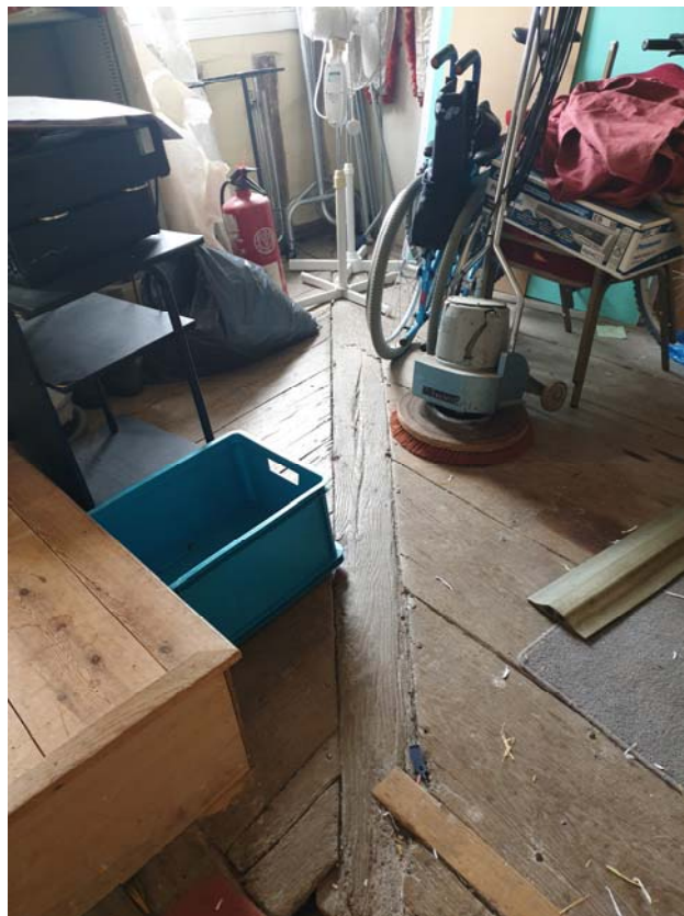
Photograph 56 – Rooms 'C5 & C6' used as a storage area
