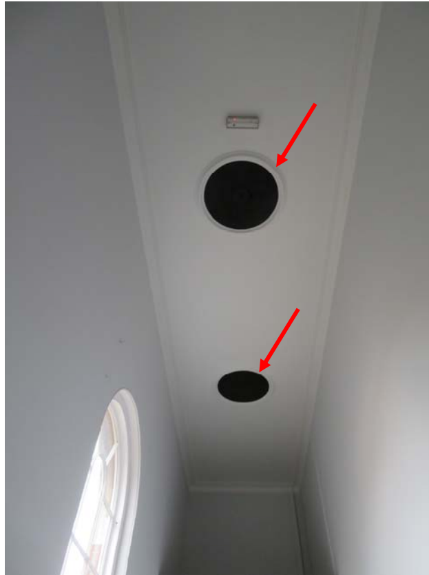
Photograph 141 – Existing grills in the ceiling noted to the stair lobby within the New Town Hall
