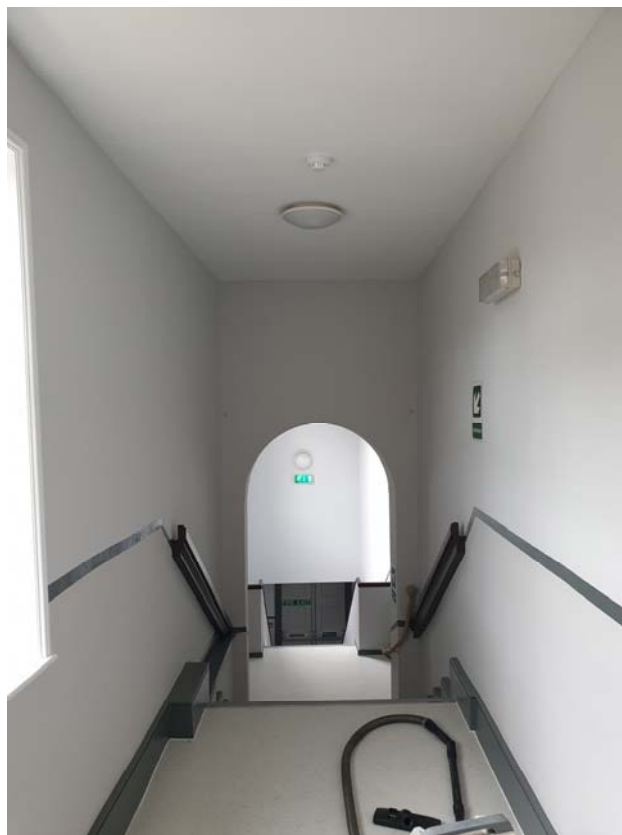
Photograph 118 – Existing Hallway linking the Old Town Hall to the New Town Hall
