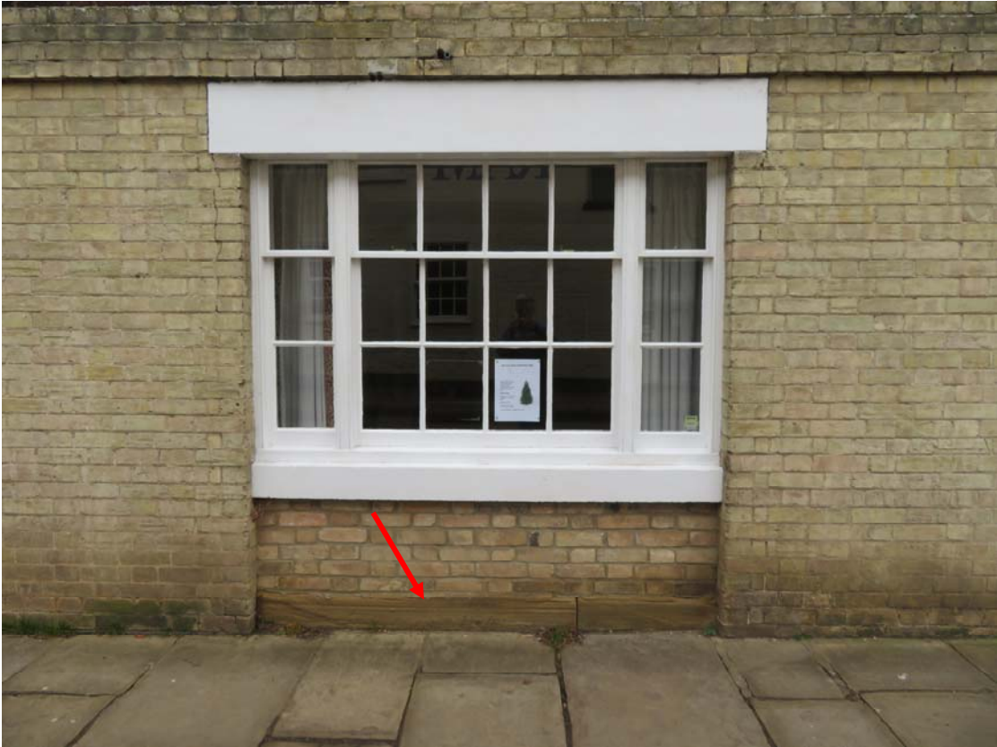
Photograph 122 – York stone paving extending out to the kerb line
