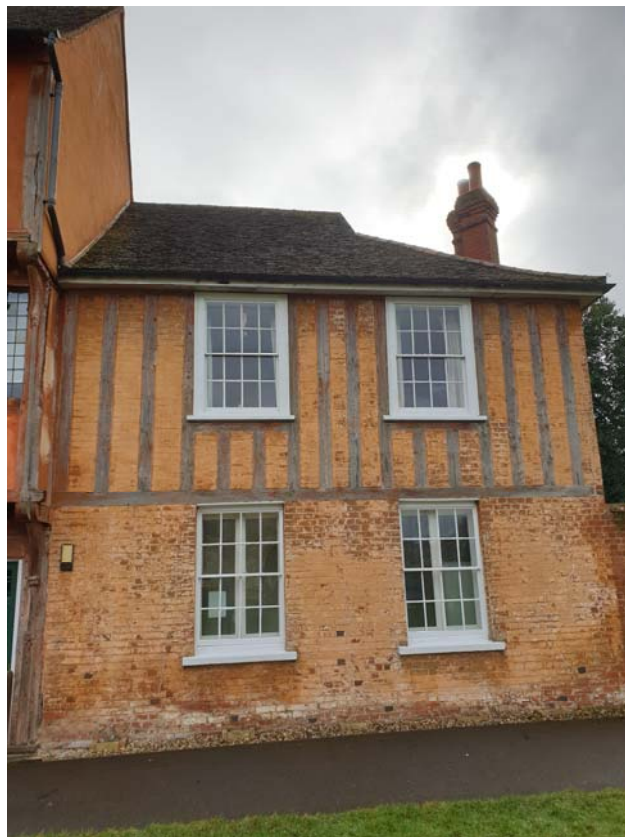
Photograph 12 – North elevation of the Market Hall's west section
