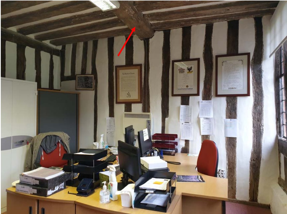
Photograph 81 – Room 'R11' and beam over
