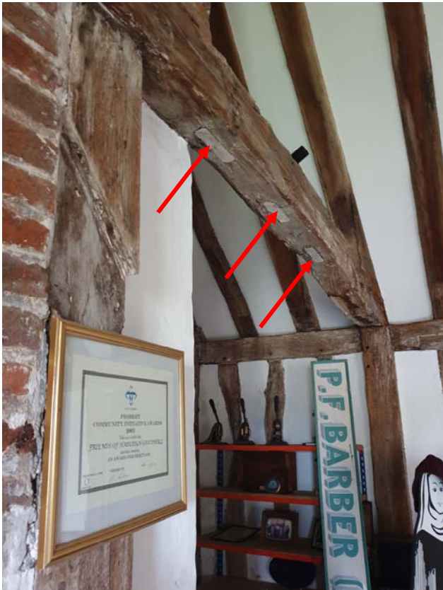
Photograph 53 – Filled mortices indicating an original partition, now removed ('C1')
