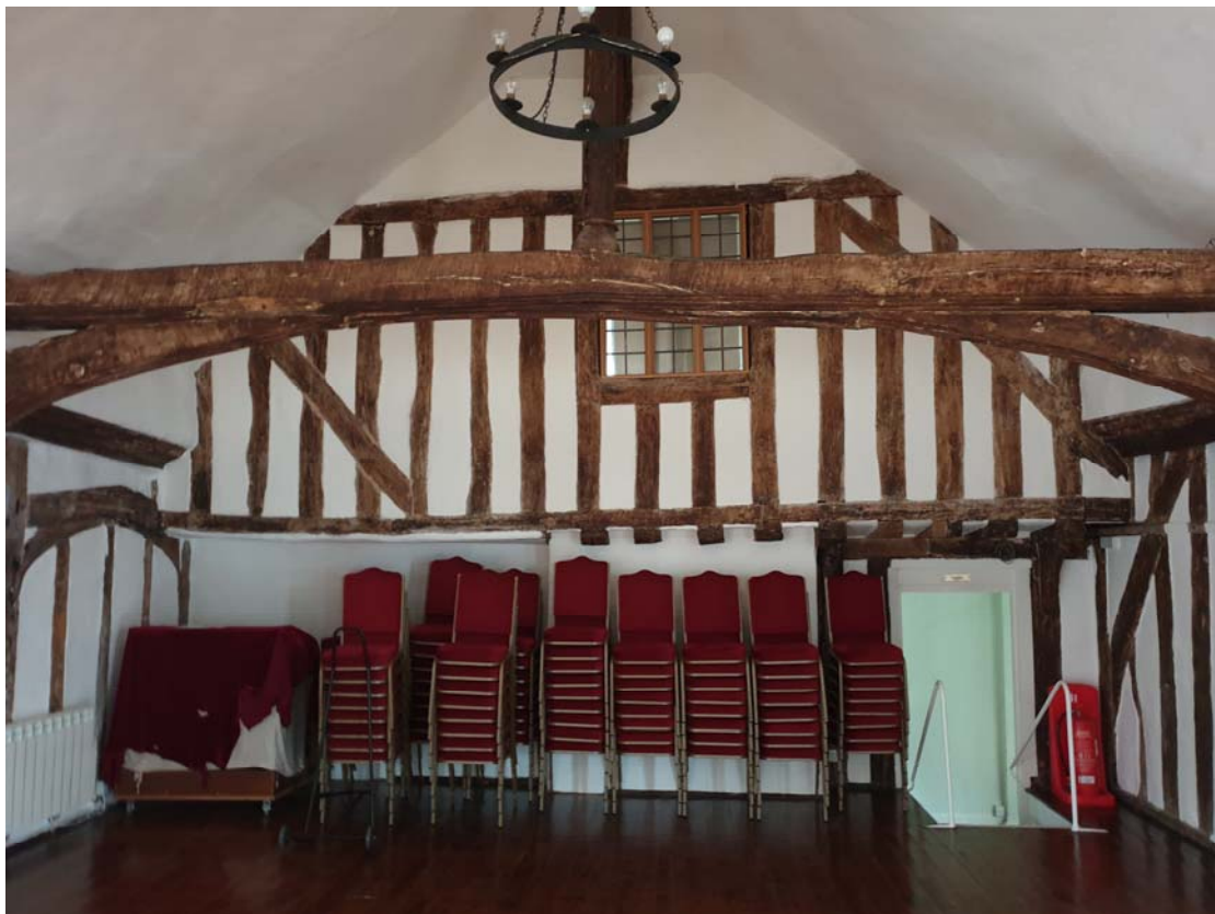
Photograph 114 – North wall of room 'L1'
