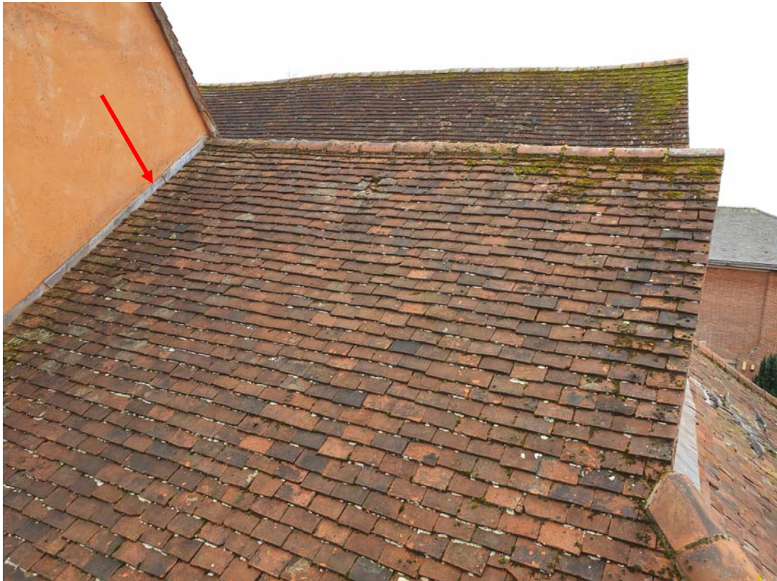
Photograph 03 – Lead flashings to the Market Hall's roof
