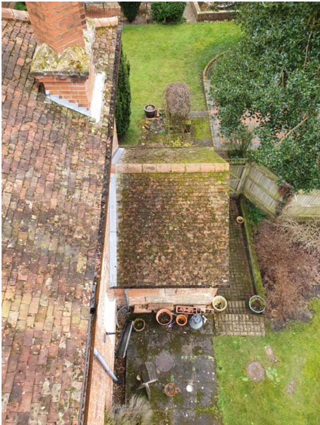
Photograph 06 – Far west roof over porch, as seen from the cherry picker
